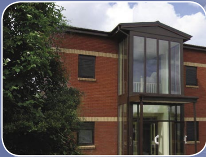
Brick clad building
